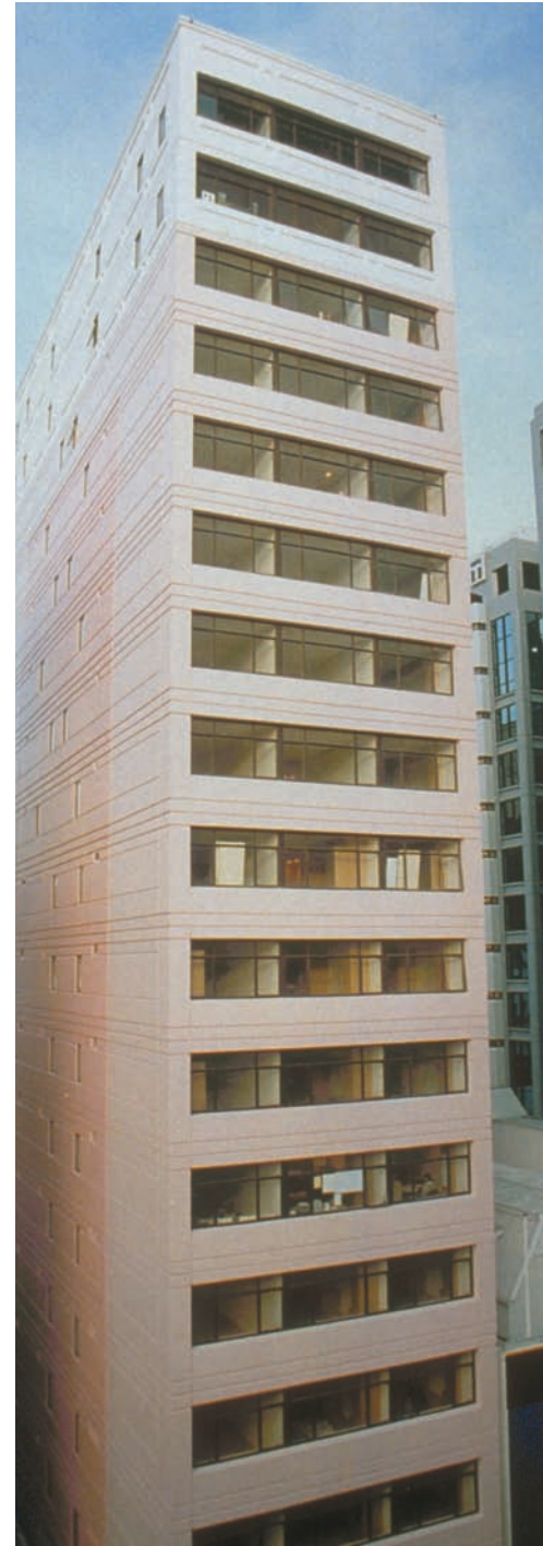
18 storey apartment building erected in 16 weeks using glass reinforced concrete panels.
