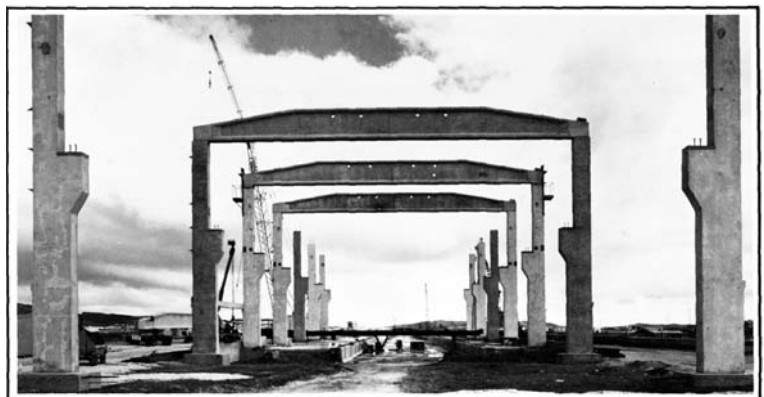
Opposite page: Precasting in New Zealand 60 years ago. A building manufactured and erected by Certified Concrete Ltd in the mid 1940s. Note the complete absence of welding and joints made at the point of contraflexure. Reinforced precast Single Tees were used as floor units (not shown).
